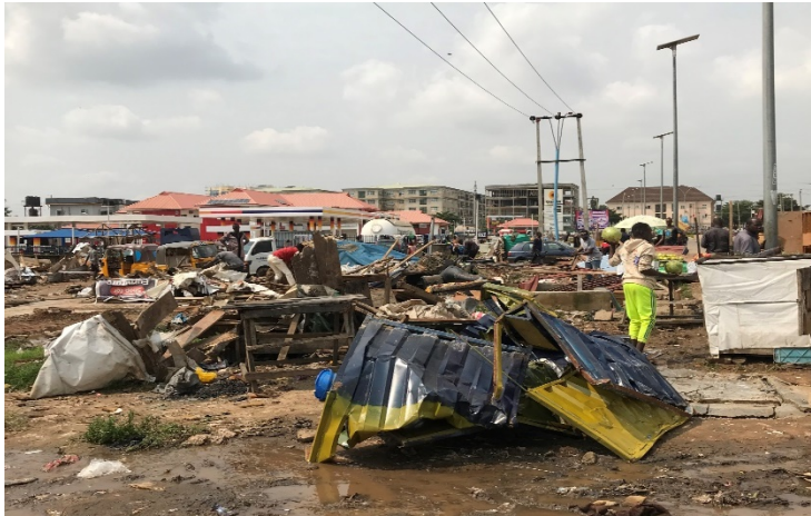
Pix 1: Scene of demolition at ....
